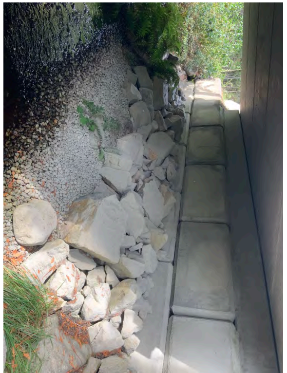
Left Bank Abutment when facing downstream
